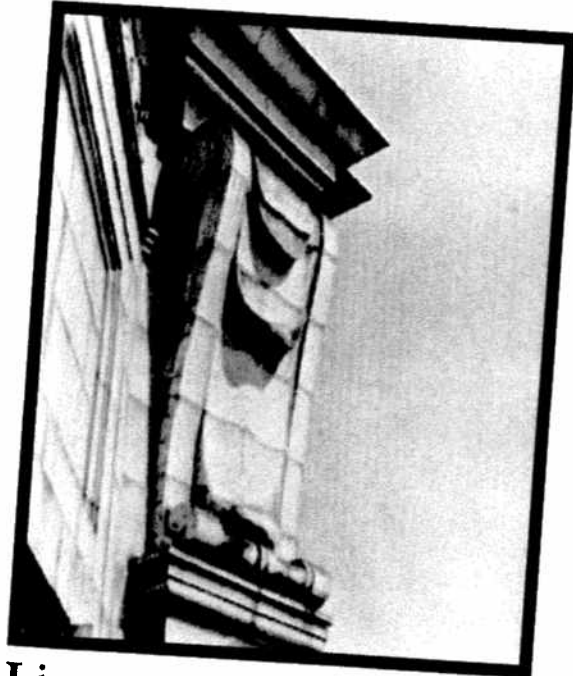
Limestone Cornice Details
