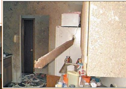
Figure B8-11. Refrigerator pierced by a 2x6. The portion of the 2x6 that is visible was 4 feet 8 inches long. It went several inches into the freezer compartment. (Oklahoma City, OK, 1999 tornado) (SOURCE: FEMA P-342)
