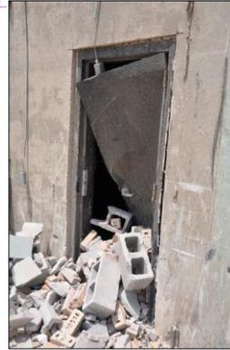
Figure B8-1. Metal door breached by wind-borne debris (this door was not designed to resist debris).
